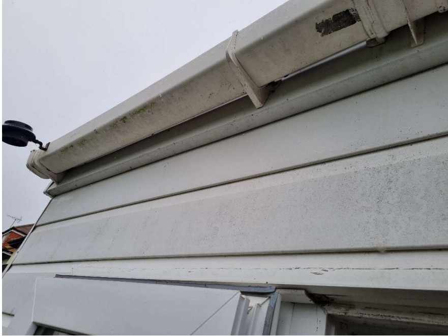
Figure 1 (Well sealed eaves to existing extension)
