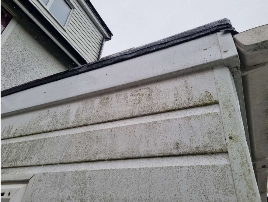
Figure 2 (Well sealed verge to existing extension)
