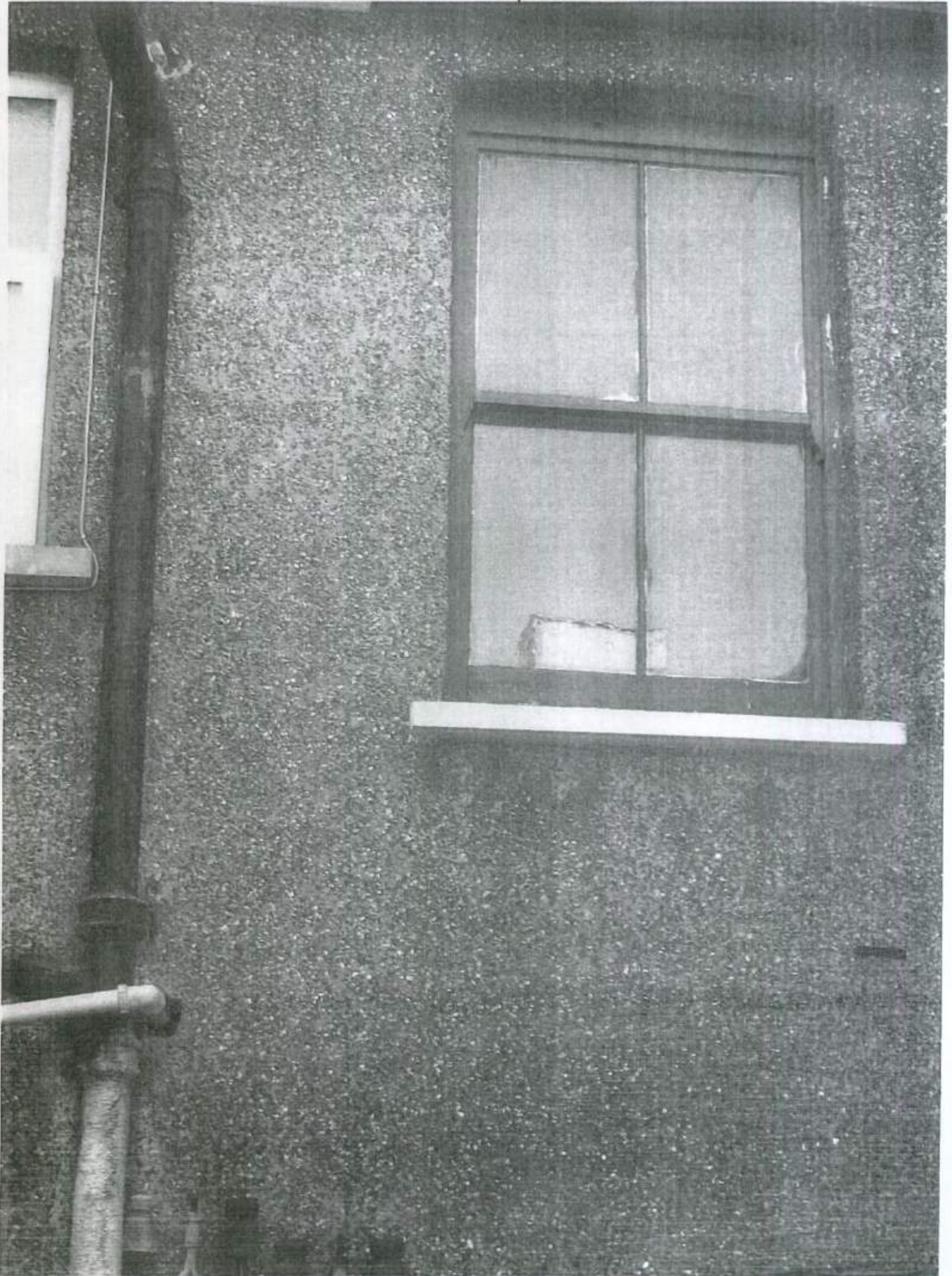
Window is Rear Bedroom Right
