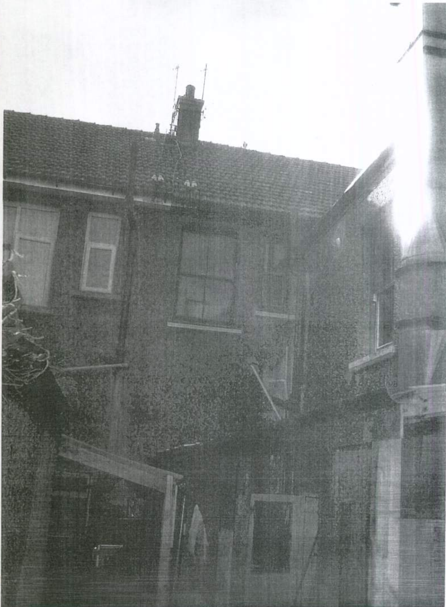
ARUN DISTRICT COUNCIL FP/184/11/ As previous page showing more clear clearly Bathroom window
