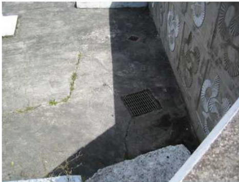
Photograph 8 – Existing surface water drainage on site to the rear of the concrete sea wall
