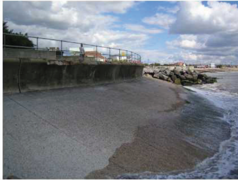
Photograph 6 – Concrete foreshore and wave return structure to the front of the site
