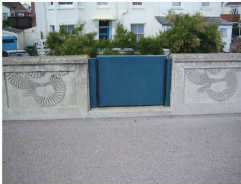
Photograph 7 – Existing floodgates through the concrete wall on the sea facing boundary
