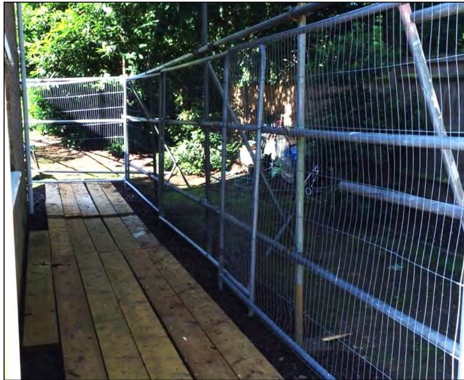
Scaffold board pedestrian ground protection
