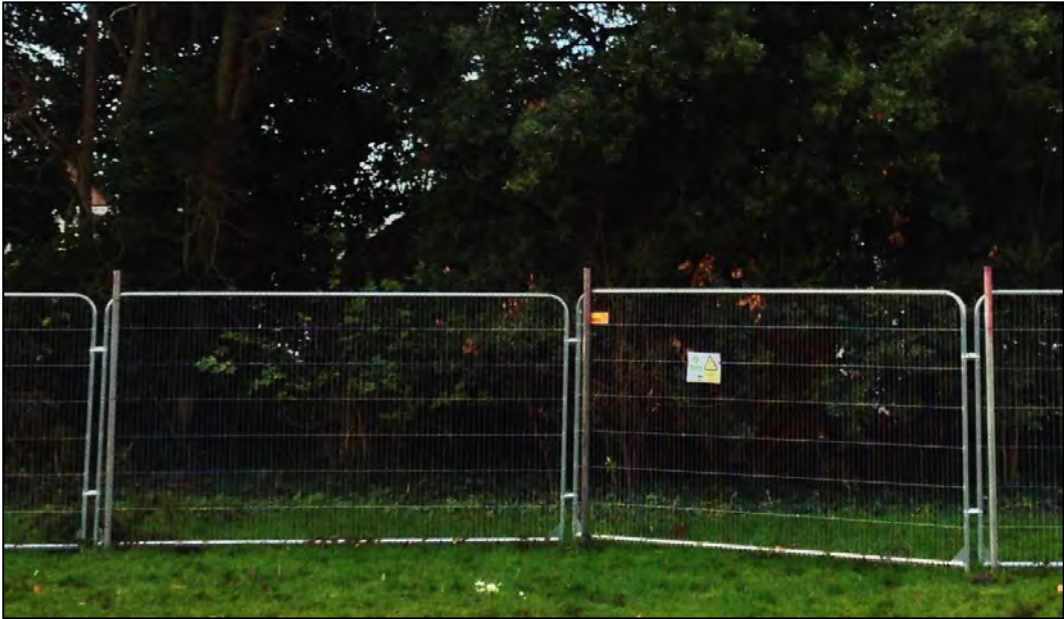
Weld-mesh panels on scaffold uprights
