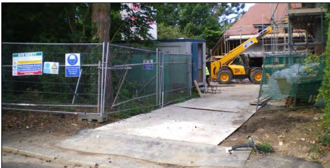
Vehicular ground protection trackway
