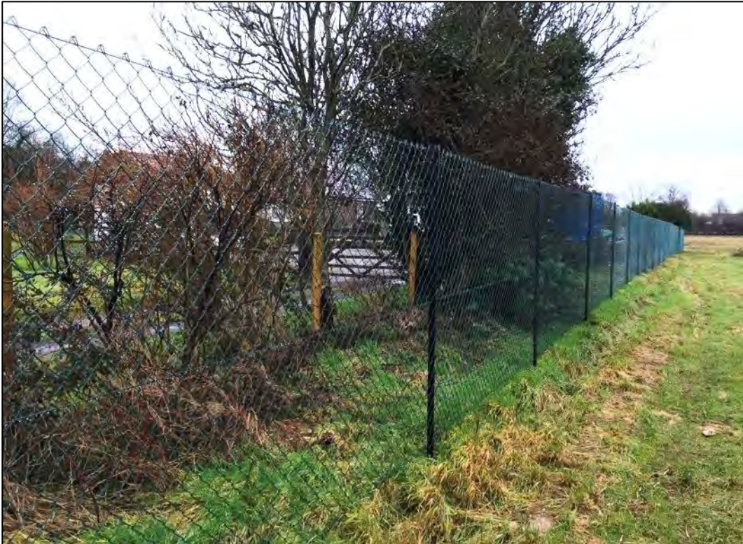
Chain-link on angle-iron uprights
