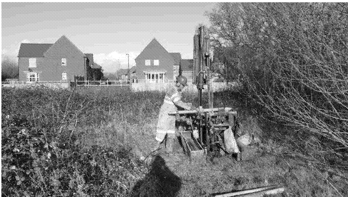
Photograph 4: Window Sampling Rig at BH5
