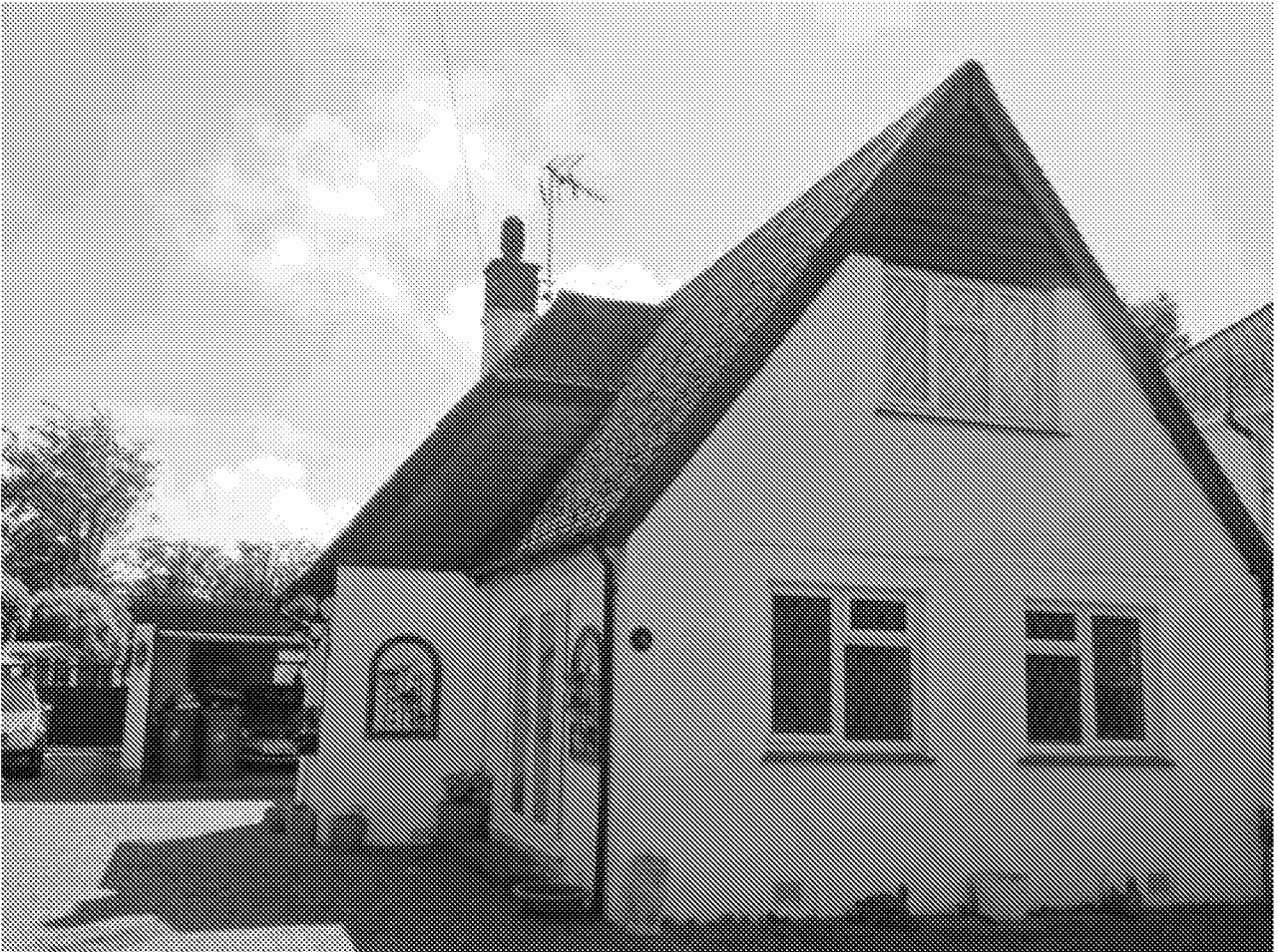
View of the North elevation
