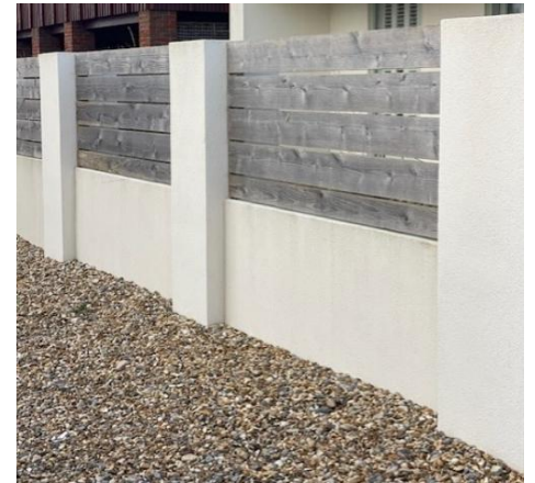
Item 4. Render Wall with Timber Infills
