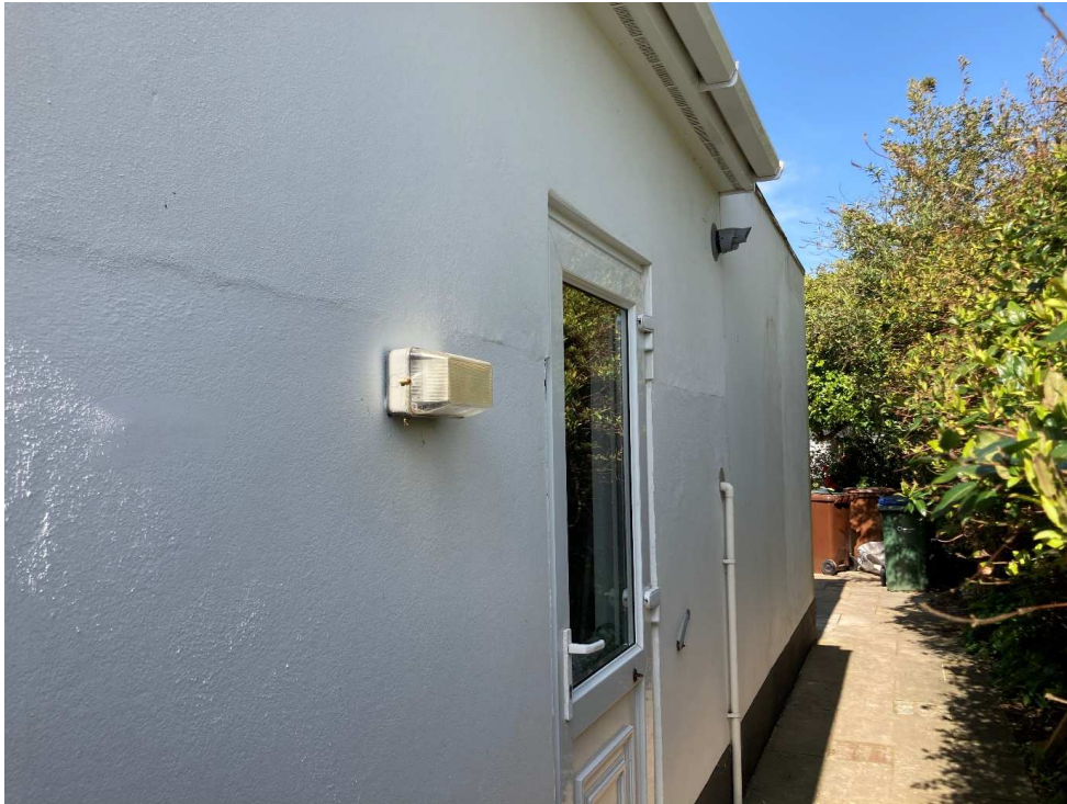
Side [East] Elevation, viewed beyond front wall
