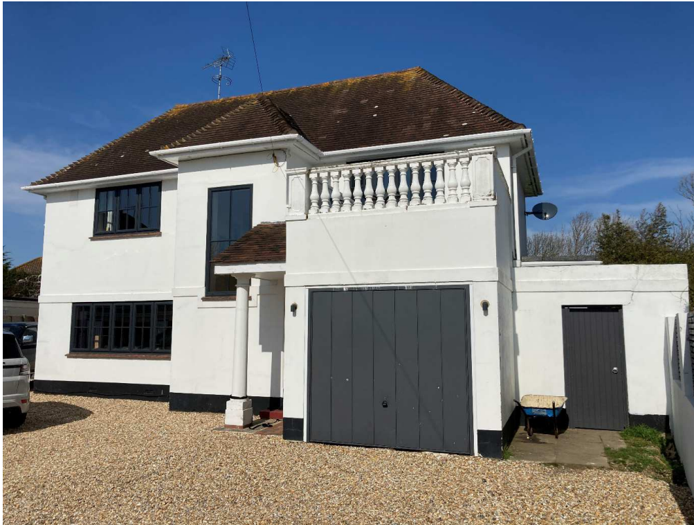
Front [North] Elevation, viewed from front driveway
