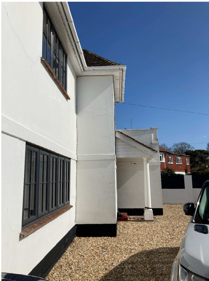
Side [West] Elevation, viewed from front driveway
