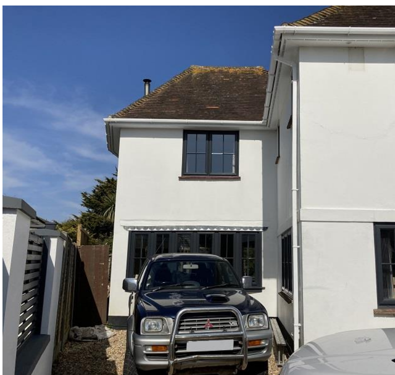
Front [North] Elevation LHS, viewed from front driveway
