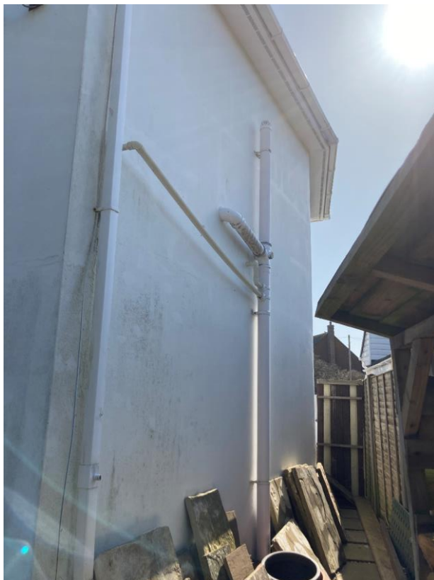
Side [West] Elevation, viewed from rear garden
