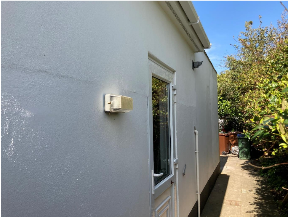
Side [East] Elevation, viewed beyond front wall
