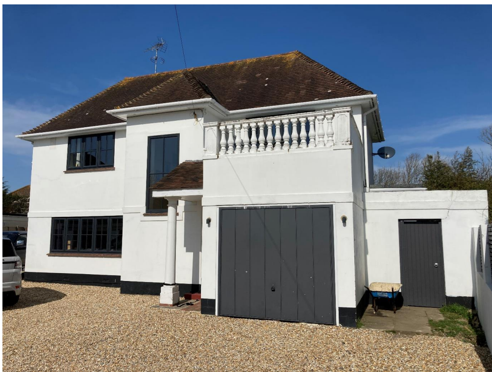
Front [North] Elevation, viewed from front driveway
