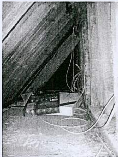
Side loft, west (front) side
