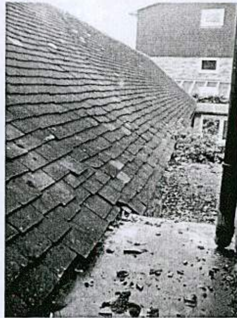
View from window over extension to east
