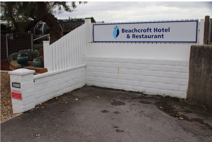
View 2 Existing Elevation from Clyde Road
