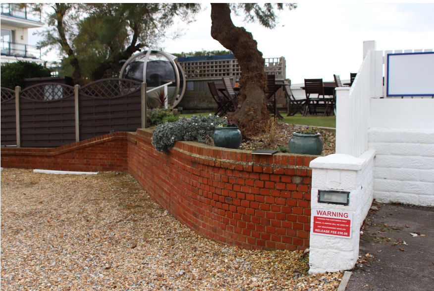
View 3 Existing Elevation from Car Park
