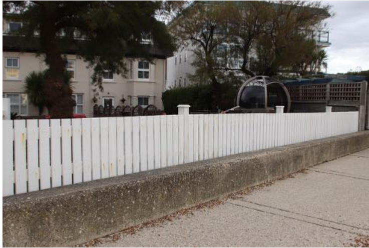
Site Photo 1 (View from the promenade)
