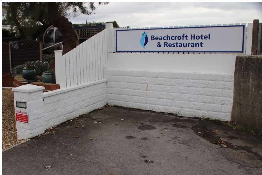
View 2 Existing Elevation from Clyde Road
