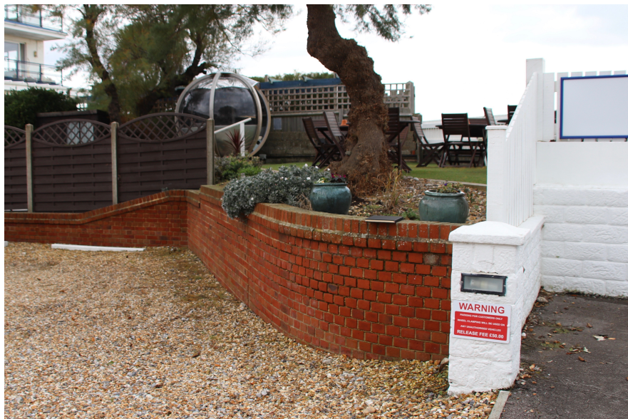
View 3 Existing Elevation from Car Park
