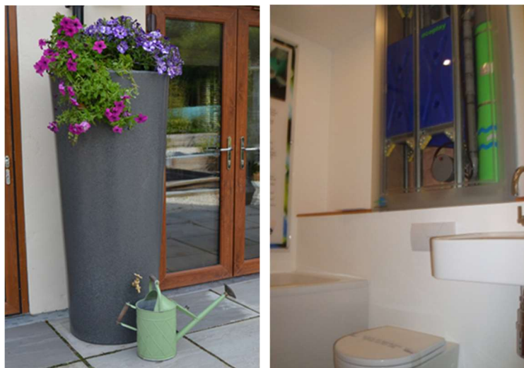
Figures 6 & 7: External rainwater harvesting butt & EcoPlay unit above WC
