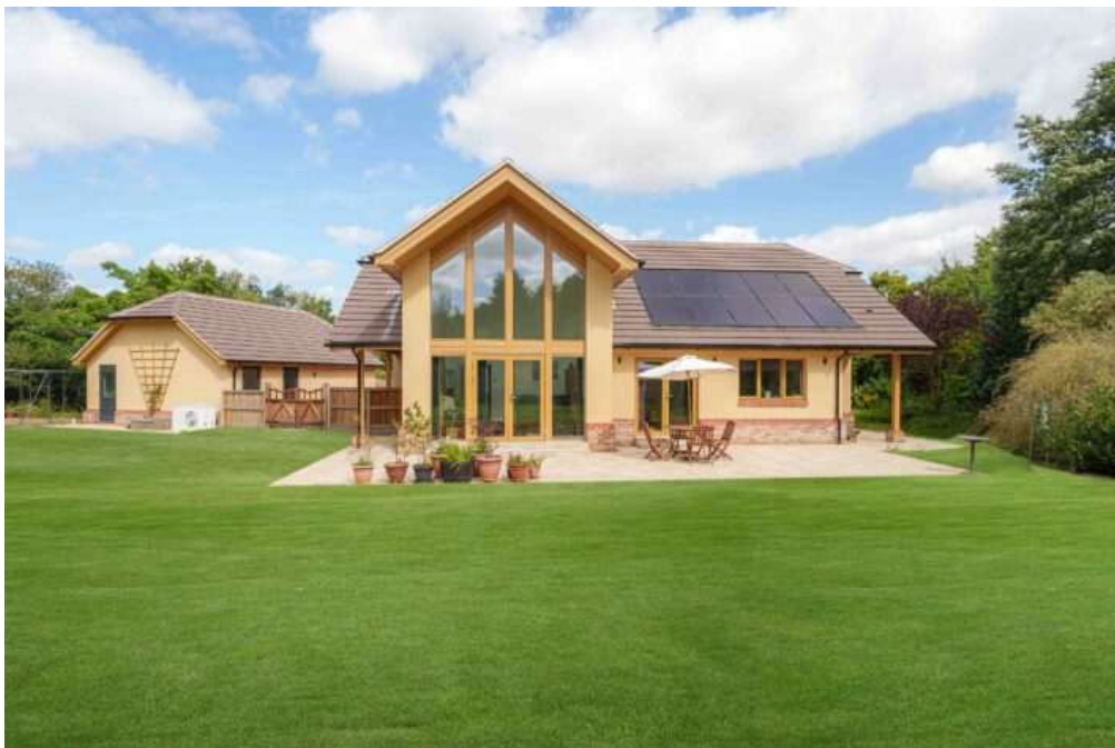
Figure 4: A Scandia-Hus house with solar PV installation
