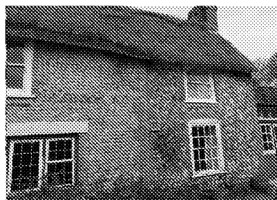
External walls of local beach cobbles and flintwork with red brick. South wall
