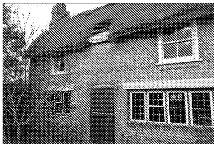
External walls of local beach cobbles and flintwork with red brick. South wall
