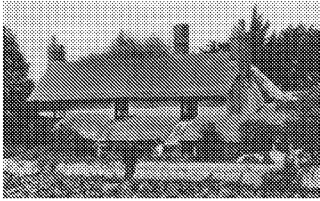
Long straw thatch with flush ridge: 1890...
