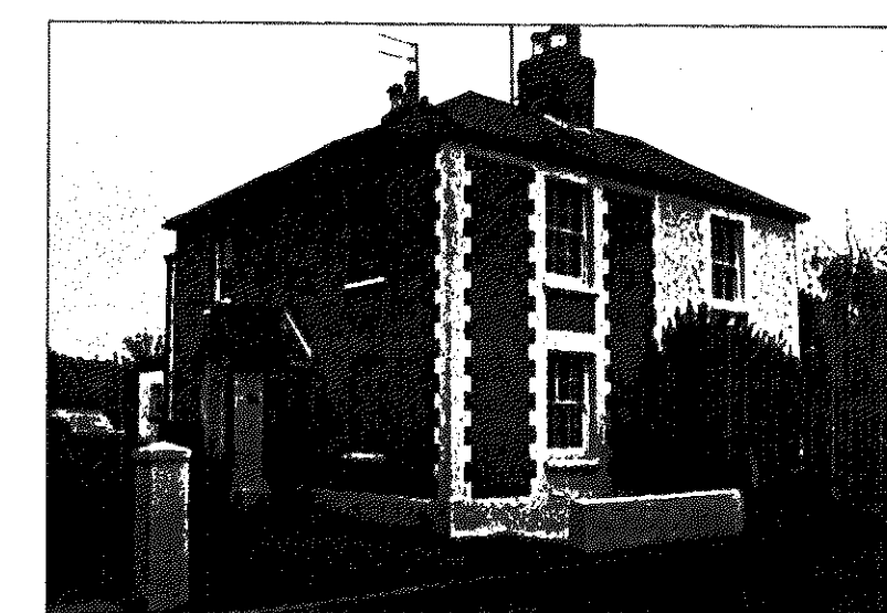
Existing Front / Side Elevation (Photograph) Scale NTS
