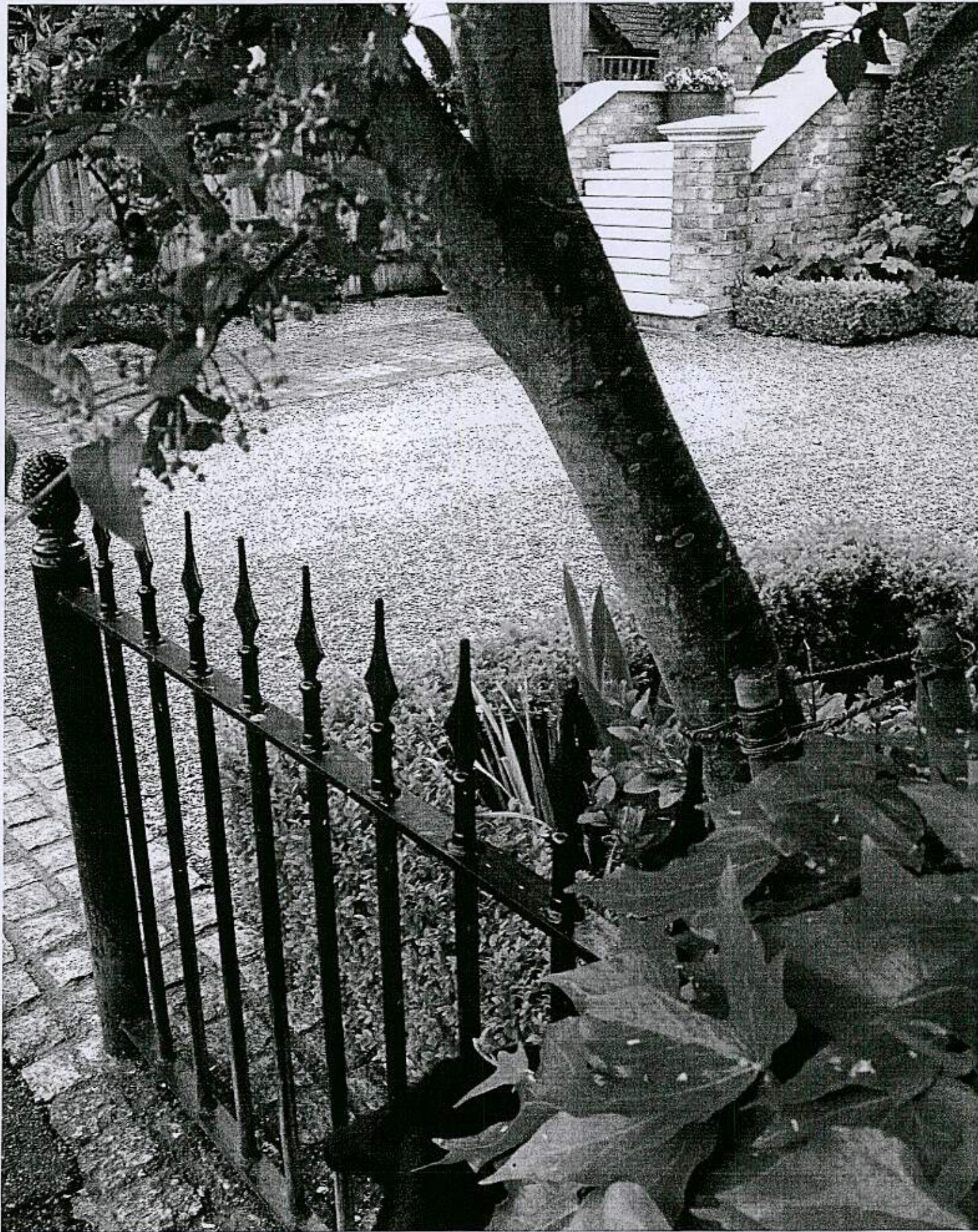
Example of gravel/stone porous 'hardstanding'
