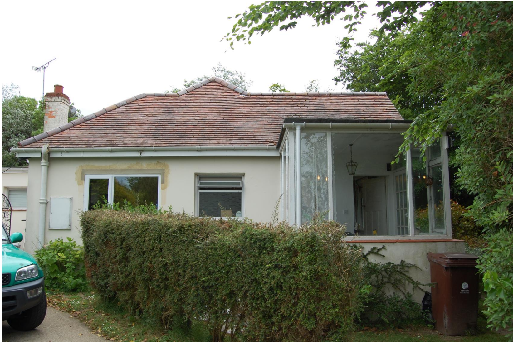
View from Upper West Drive
