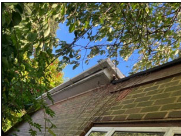
Photograph 20 the northern face of the house is well sealed and intact
