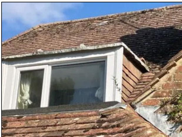
Photograph 18 Hanging tiles on the west-facing dormer window
