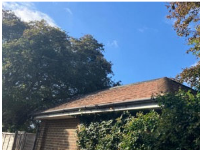
Photograph 31 southern view of the garage at 42 Sea Lane
