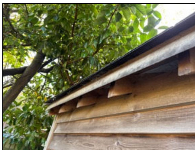
Photograph 33 gaps at the eaves of the carport leading into the structure. the wooden cladding is very well sealed and free from gaps
