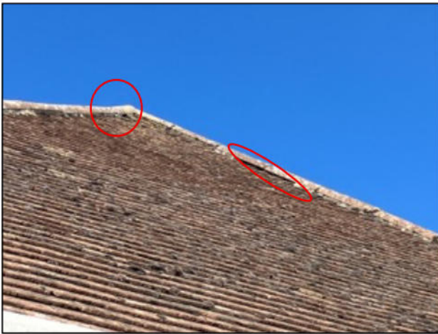
Photograph 14 PRFs at the ridge of the south-facing roof pitch
