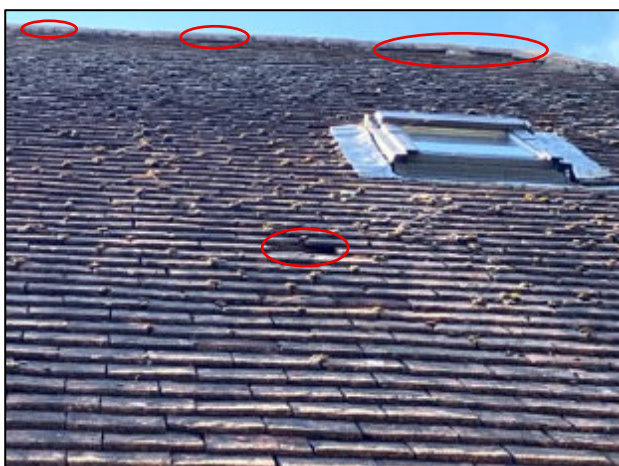
Photograph 22 PRFs on the east-facing roof pitch
