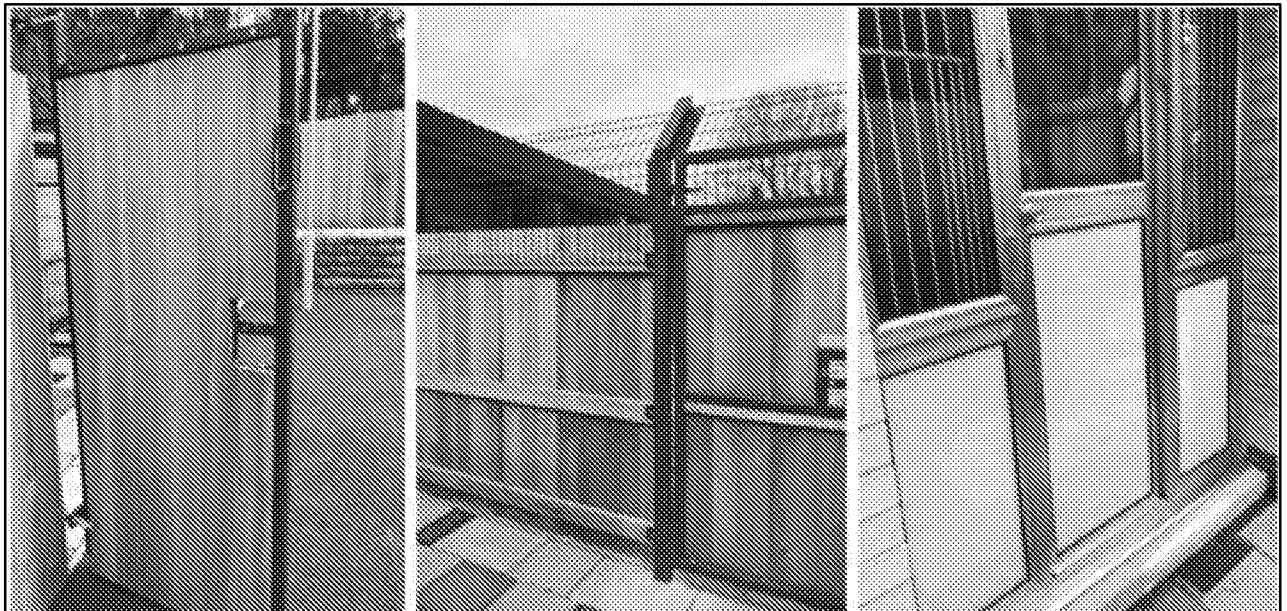
Figure 4. External Exercise Areas and External Kennel doors
