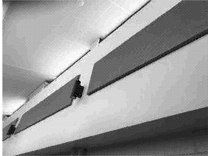
Figure 5. Internal Wall Mounted Absorber Panels
