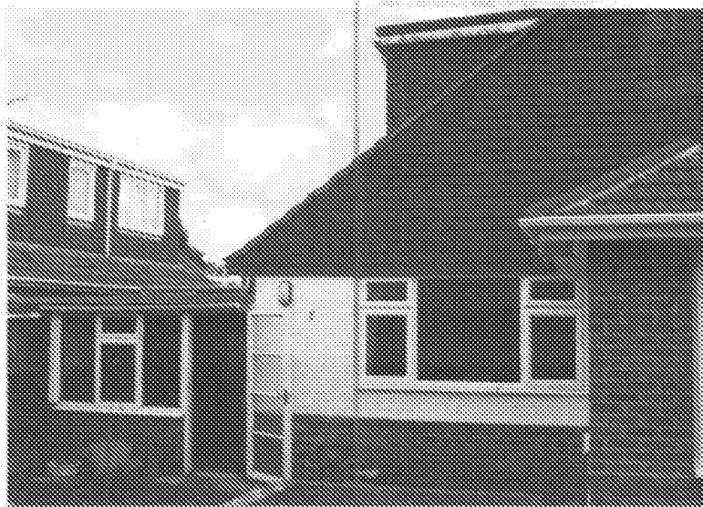
REAR (LEFT SIDE) (NORTH)
