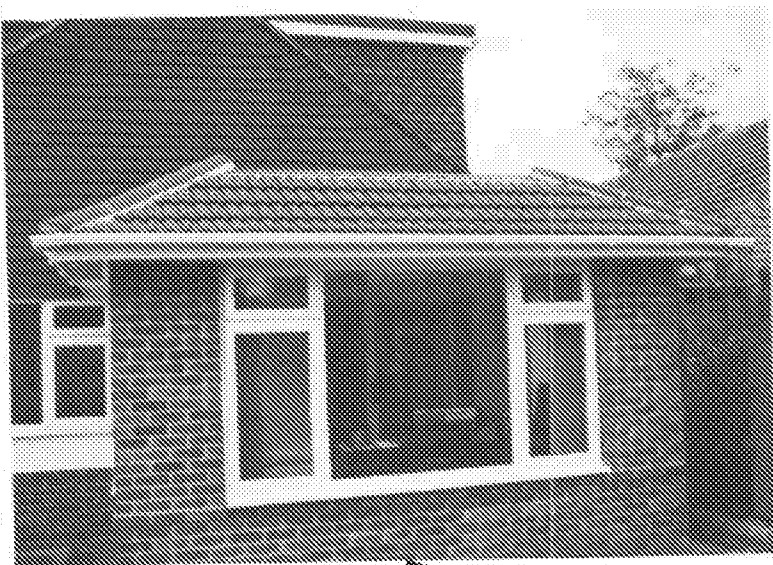
REAR (RIGHT SIDE) (NORTH)
