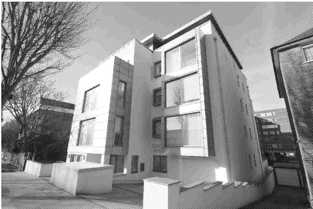
Above: Flats in Palmeira Avenue, Hove
