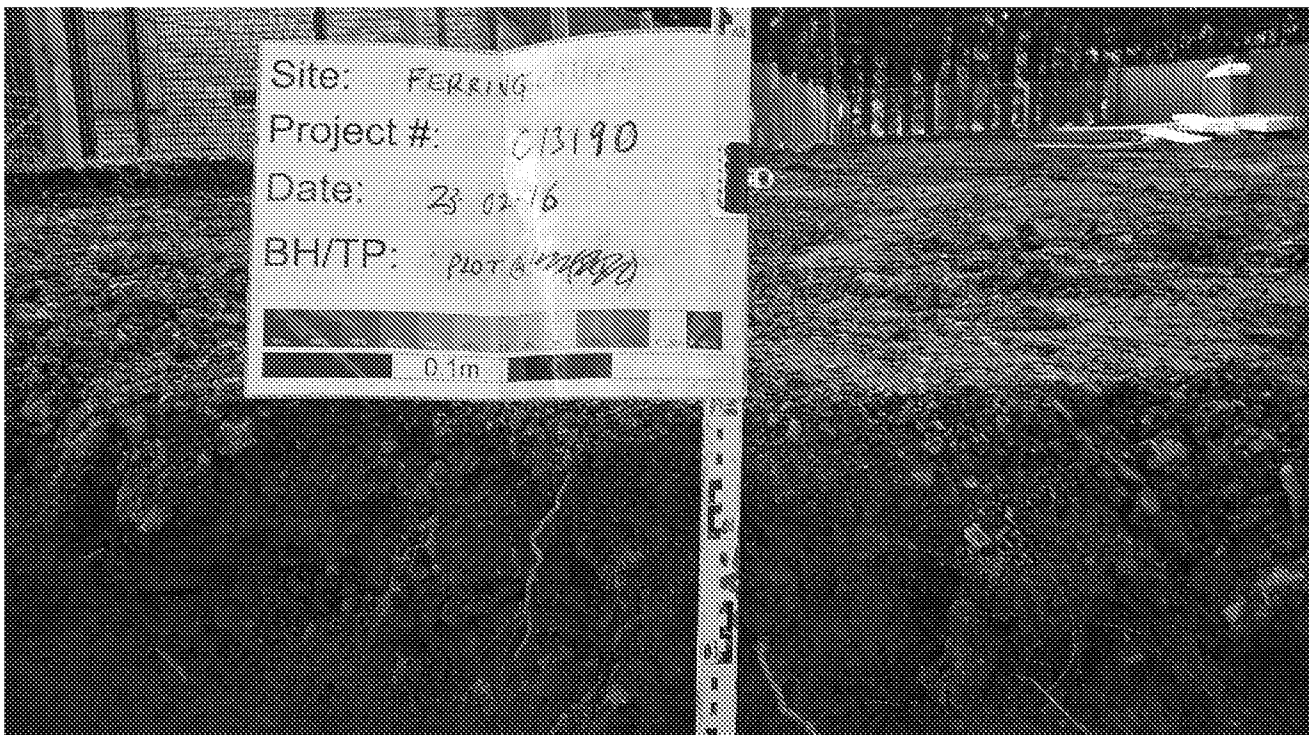
Photograph showing Area A removal depth of 0.5 metres
