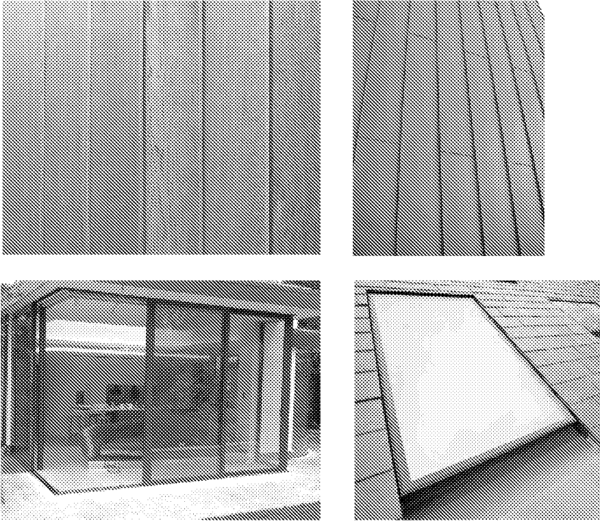
Fig 11. Materials – Timber cladding, standing seam zinc, aluminium sliding doors and flush fitting rooflights
