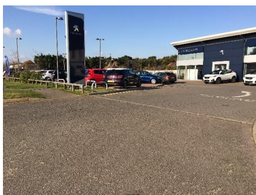
Photograph 1: Existing 'In' Access
