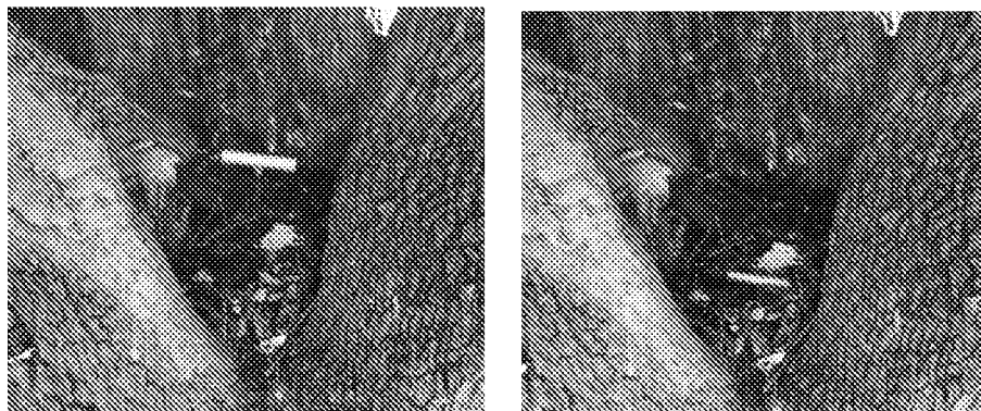
Picture 11 and 12 above showing depth of steel probe into main stem cavity.
