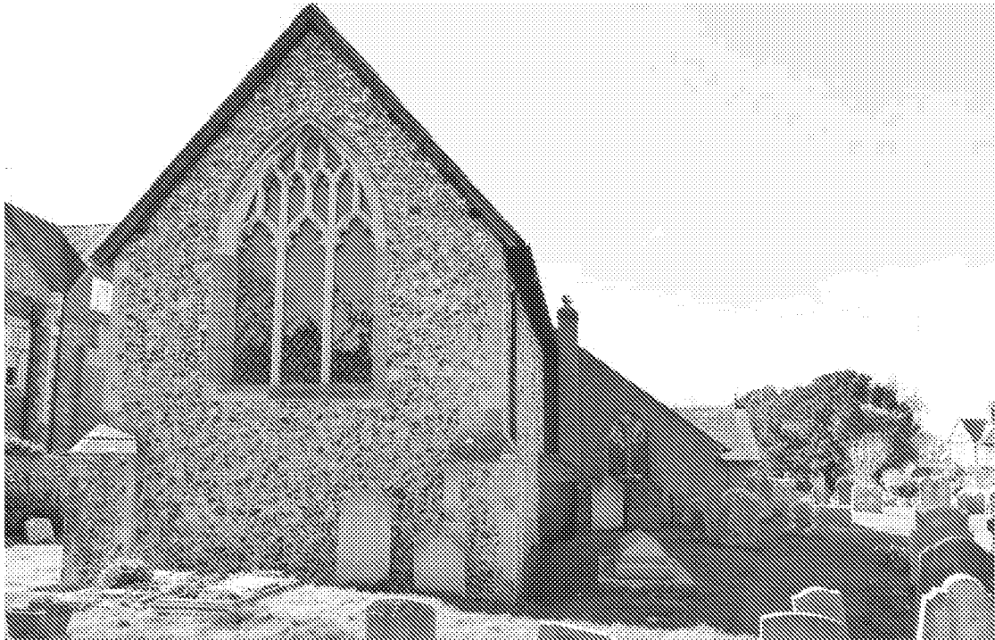
The east window to the north aisle is in the pebbledashed area of walling to the right of the boiler chimney
