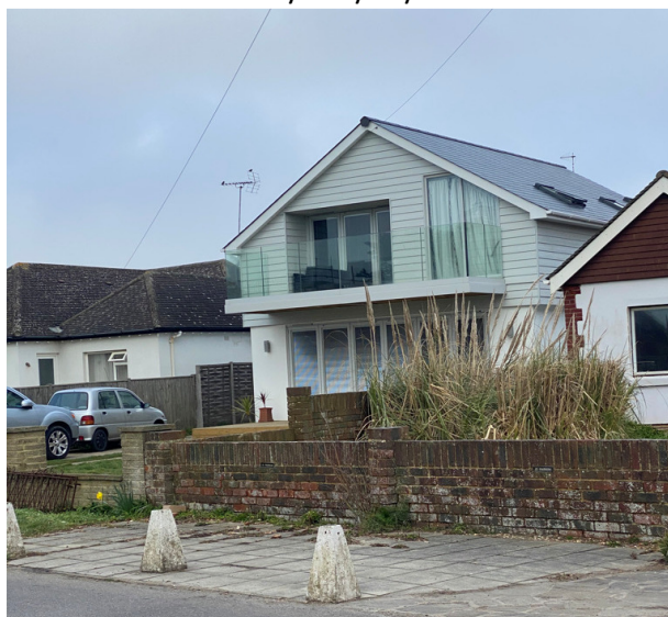
12 South Drive – FG/107/17/HH - Front elevation and balcony
