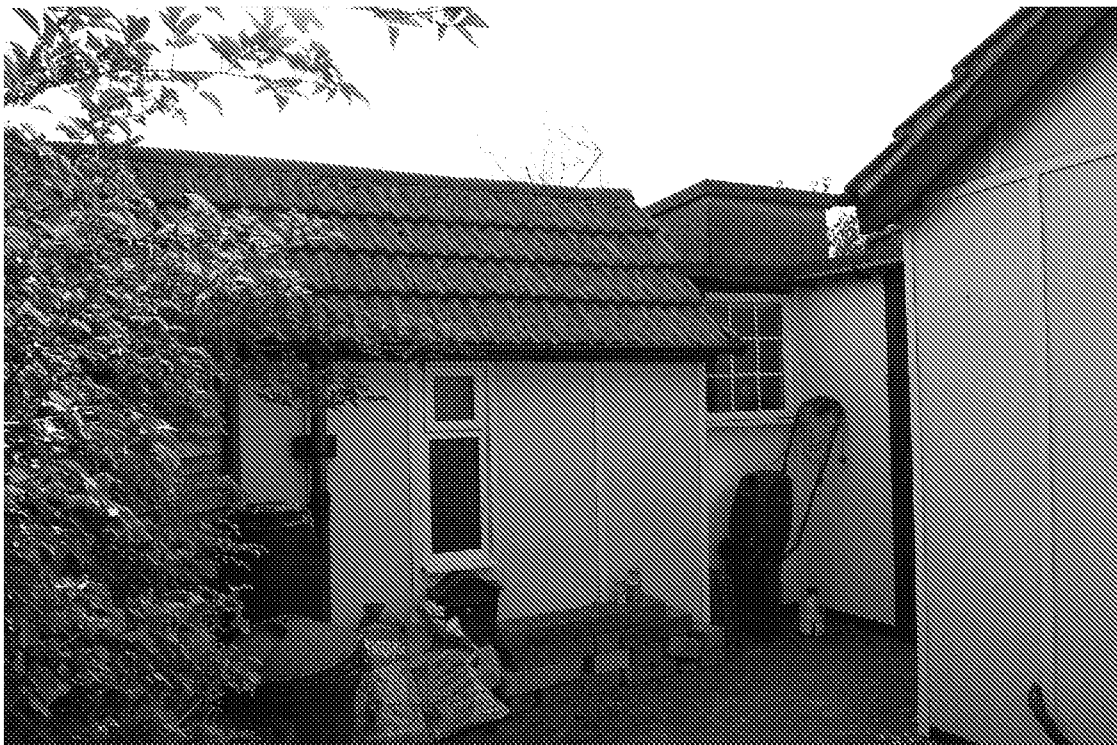
Side View Towards Rear From Driveway
