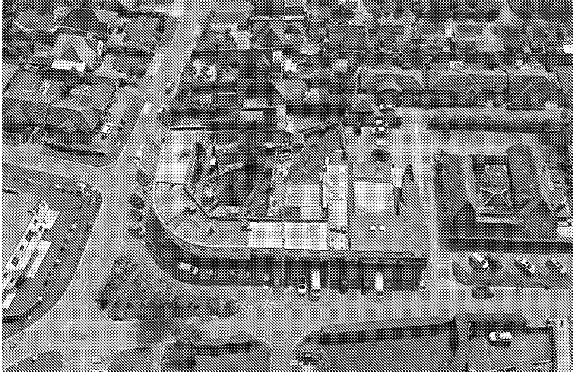
Aerial View - Google Earth 2021
