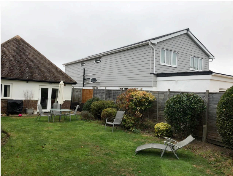
View of 9 Ocean Drive from rear [East]
