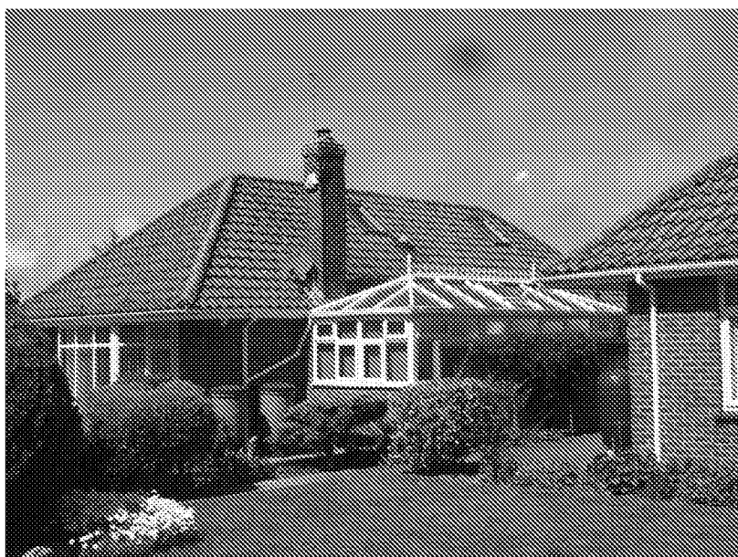
Photo 19. 40 Midhurst Drive – clear glass openable velux windows.
