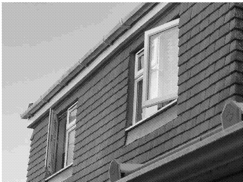
Photo 8. 61 Midhurst Drive – large dormer with side facing clear glass openable windows.
