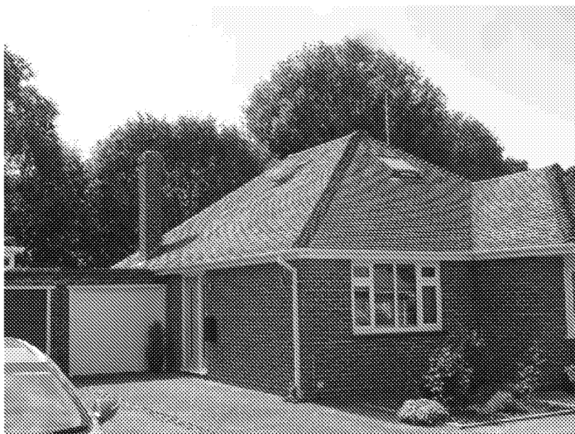
Photo 11. 57 Midhurst Drive – clear glass openable velux windows.
