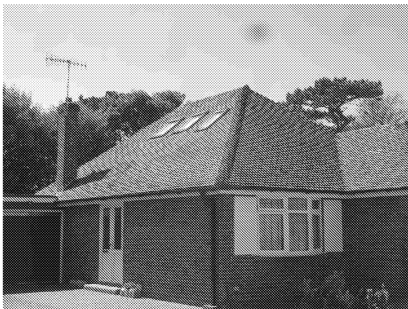
Photo 15. 45 Midhurst Drive – clear glass openable velux windows.
