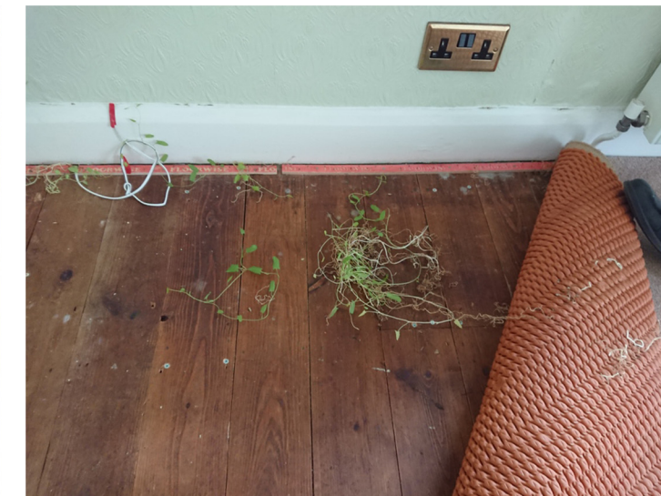
Existing condition of floors
