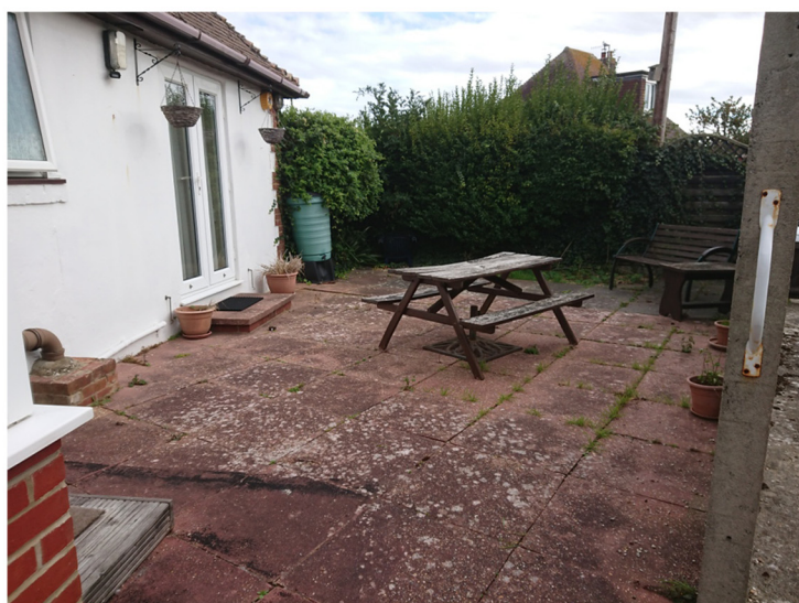
Existing front concrete paved area
