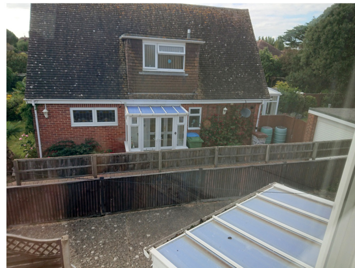
Existing view from bedroom 2 side dormer
