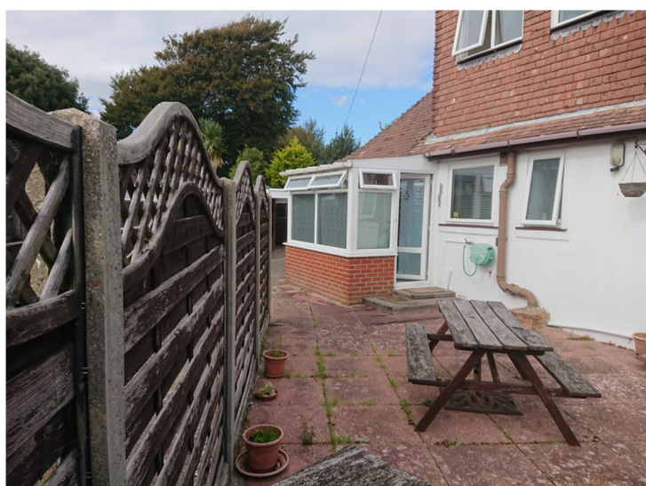
Existing front concrete paved area
