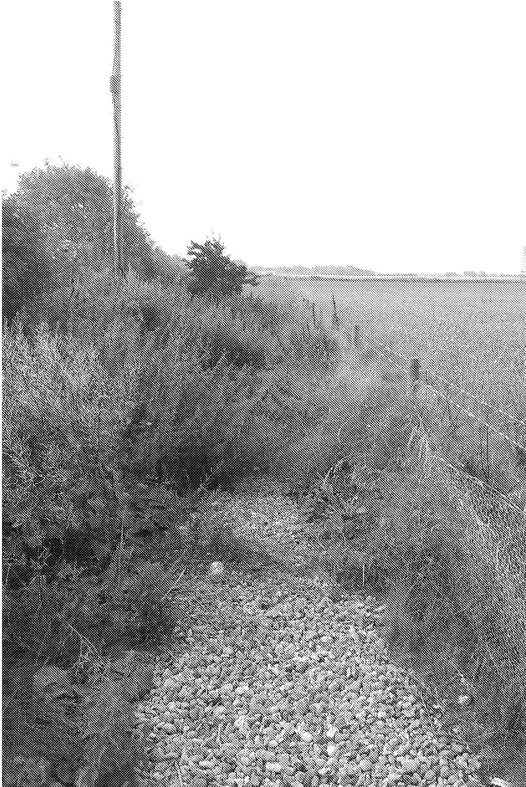
Photograph 4 – Looking south along the western boundary of the site showing the French drain which intersects any runoff from the agricultural land to the west
