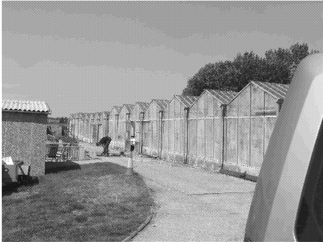
Photo 1: The existing nursery glasshouses showing drainage.
