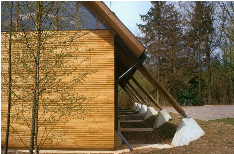
Sweet chestnut rain screen cladding at the Woodland Enterprise Centre, Flimwell
