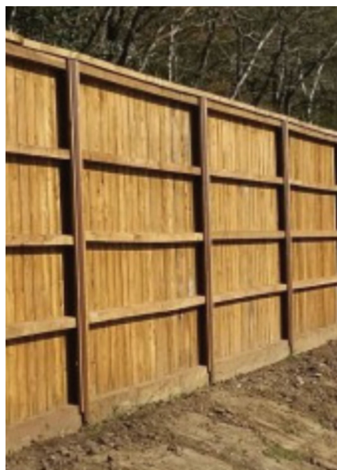
rear view of 1800mm height fence
