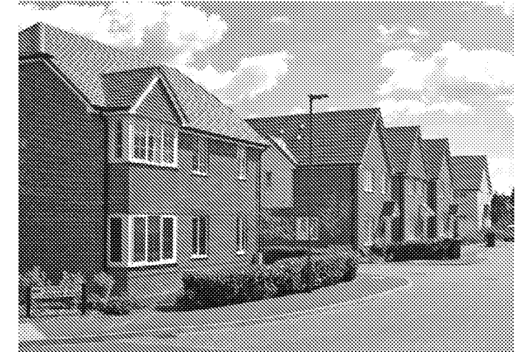
8. Two storey dwelling in brick
