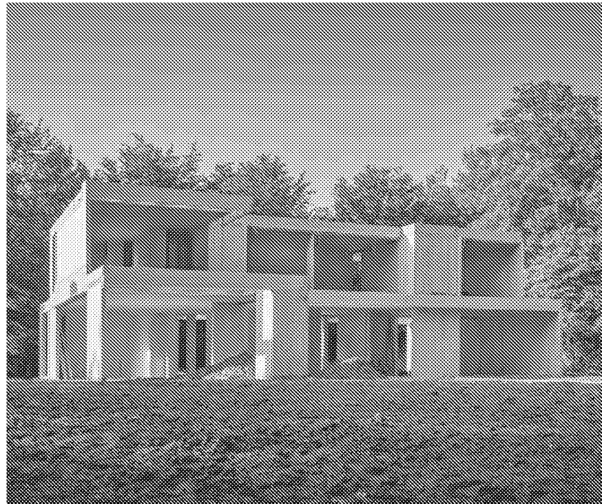
Example of a building under construction using Structural Insulated Panels
