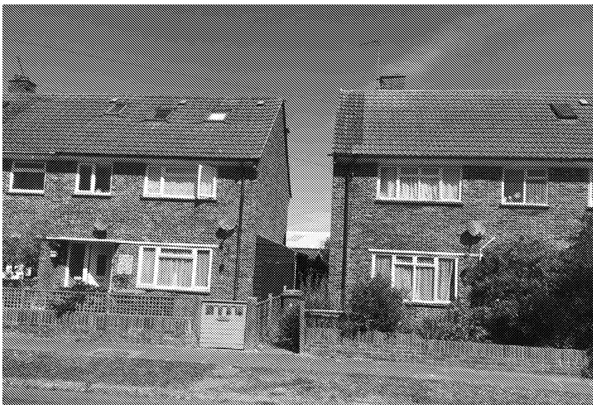
7. View through Gap between Nos 8 and 10 Meadow Way
