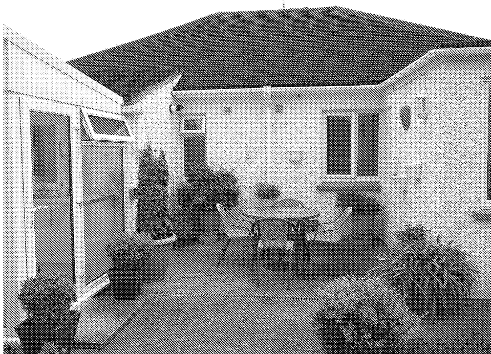
Figure 5 – Existing main house north elevation
