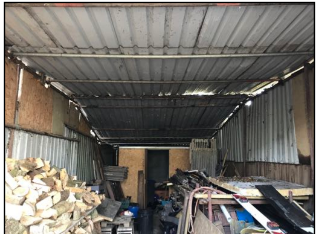
Image 4: Another example of one of the buildings constructed with corrugated material
