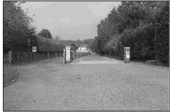
Photo 2: The access drive, facing north
