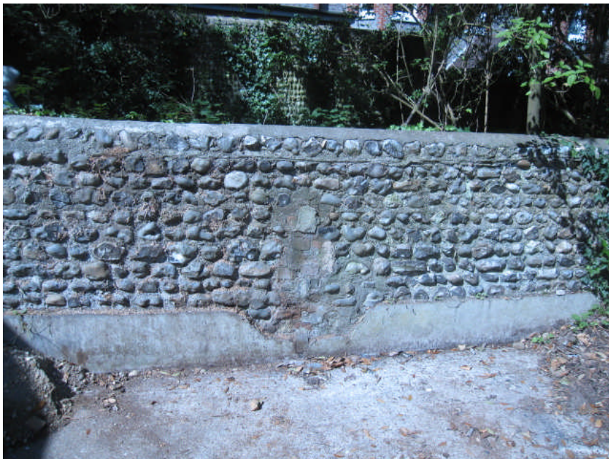
2.3 Photo 4 –North Boundary wall with evidence of a previous building's ventilation apertures
