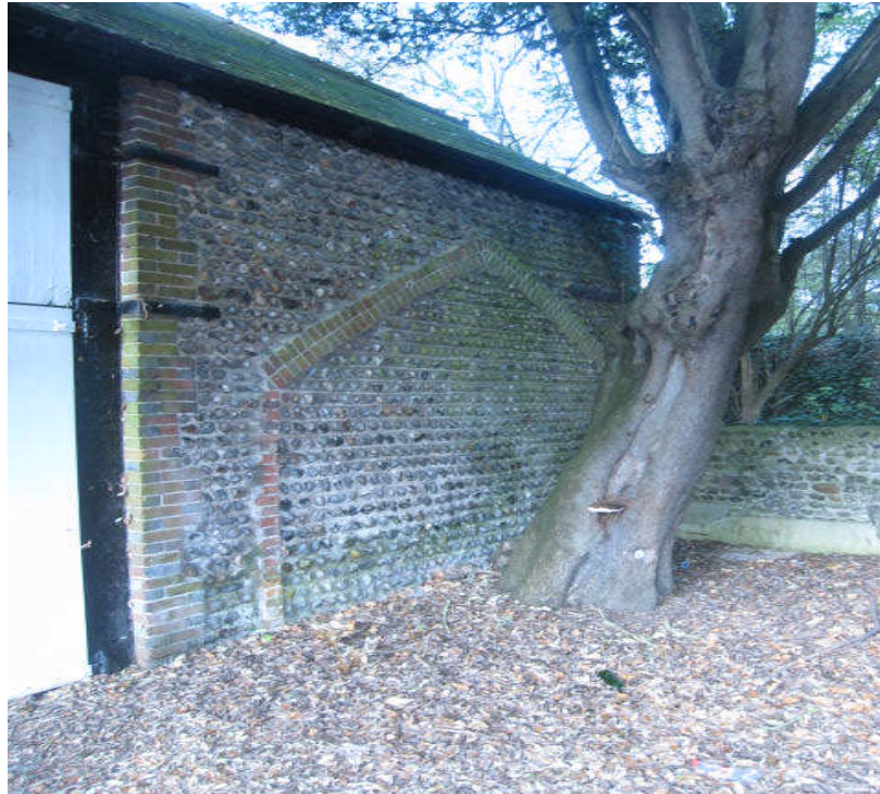
1.1 Photo 1 – The Old Barn – Northeast Elevation – Evidence of a previous building connecting to the Old Barn
