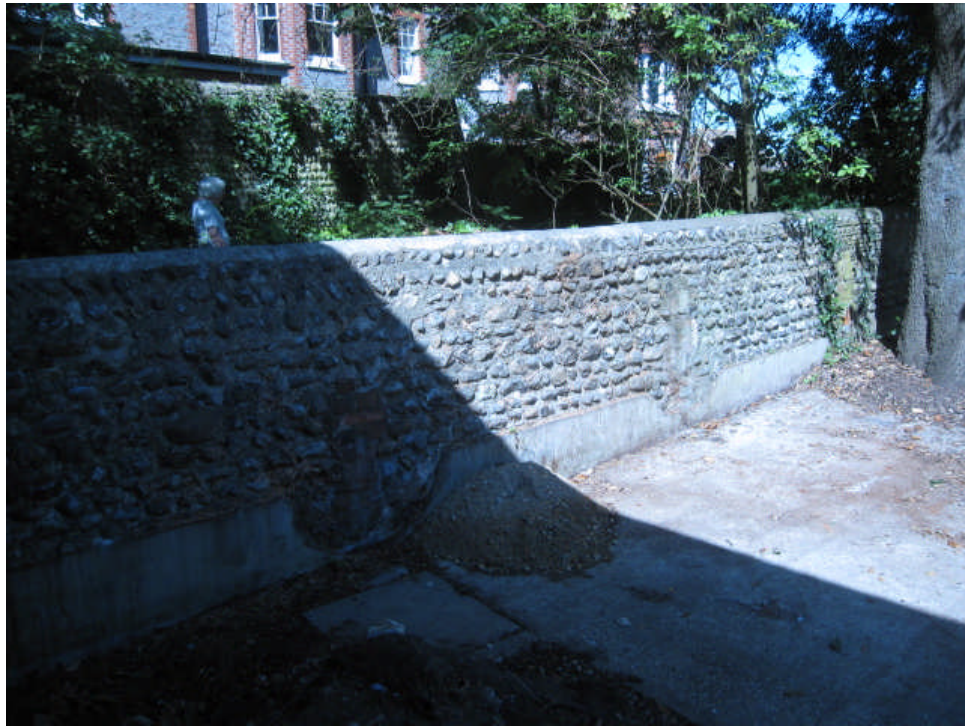
2.4 Photo 5 - North Boundary wall with evidence of a previous building's ventilation apertures
