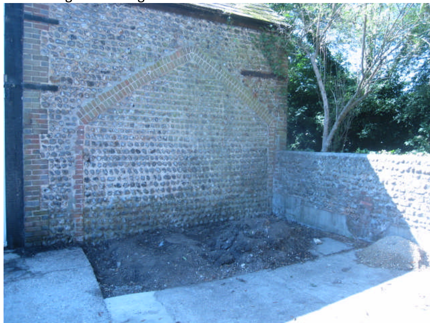
1.2 Photo 2 – The Old Barn – Northeast Elevation with tree removed – Evidence of a previous building connecting to the Old Barn
