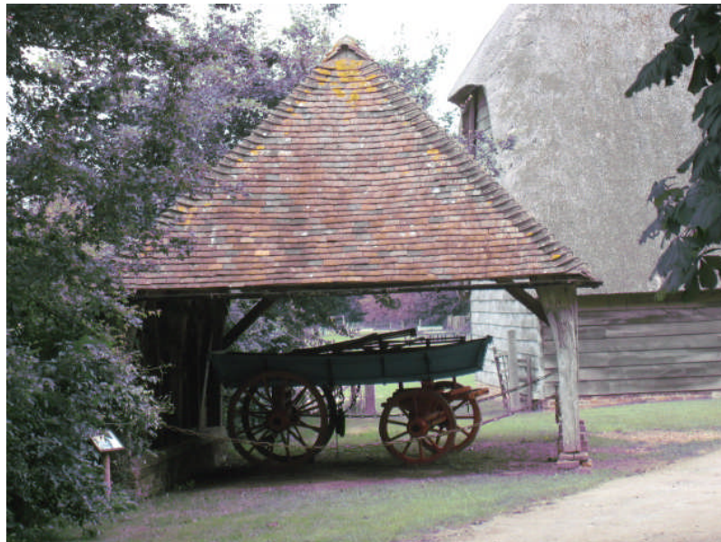
3.1 Photo 6 – Cart Shelter 1 – Side View
