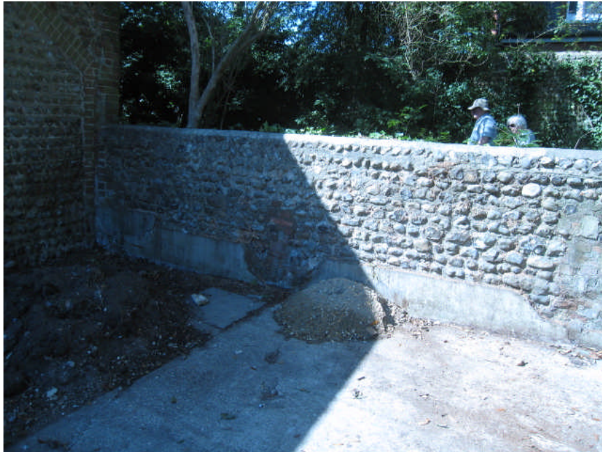
2.2 Photo 3 – North Boundary wall with evidence of a previous building's ventilation apertures
