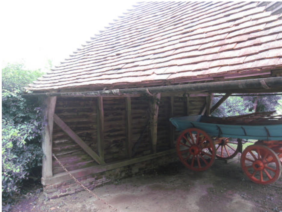
3.3 Photo 8 – Cart Shelter 1 – Internal view
