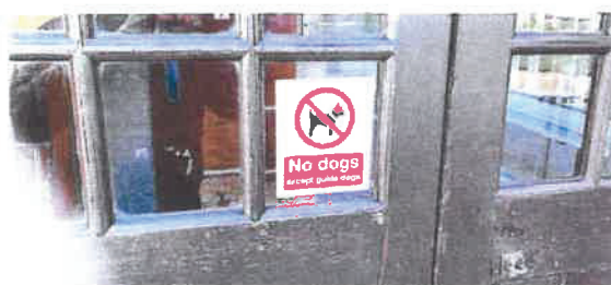
TO BE REPLACED WITH NEW
