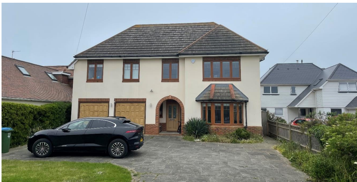
Figure 2 - Photograph of Existing Dwelling Front Elevation
