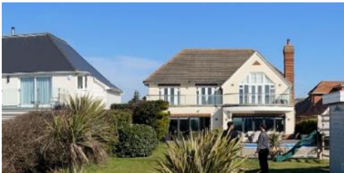
Figure 22 - Photograph of Rear of Existing Dwelling
