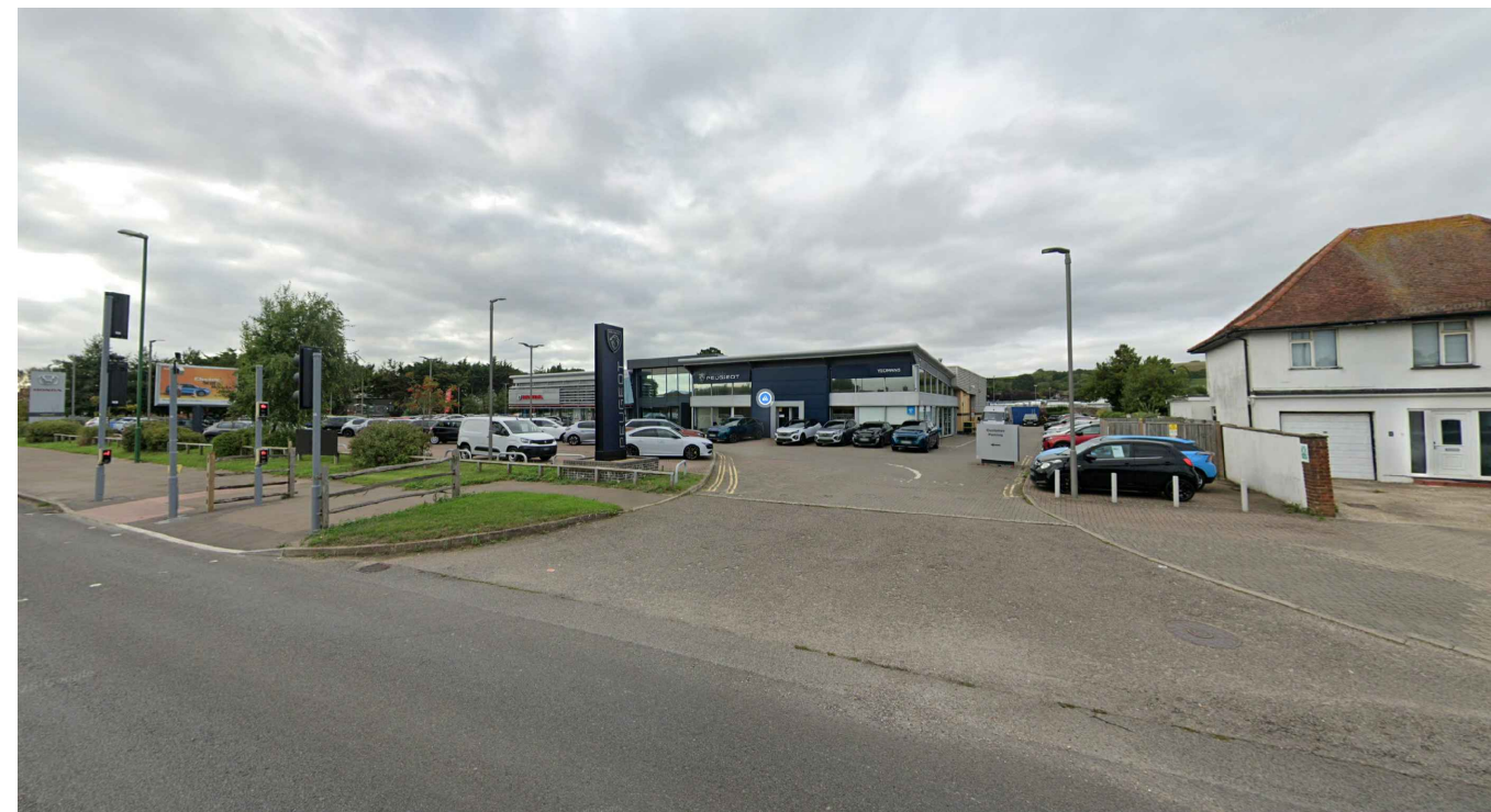
Image 4.0 View from Littlehampton Road (East Side)
