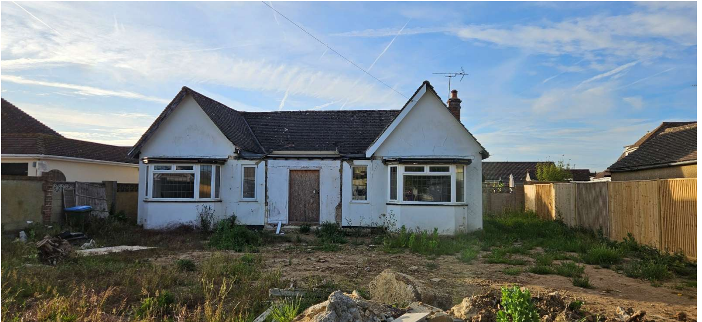
Photo 1 – Front of the building (Southern Elevation)
