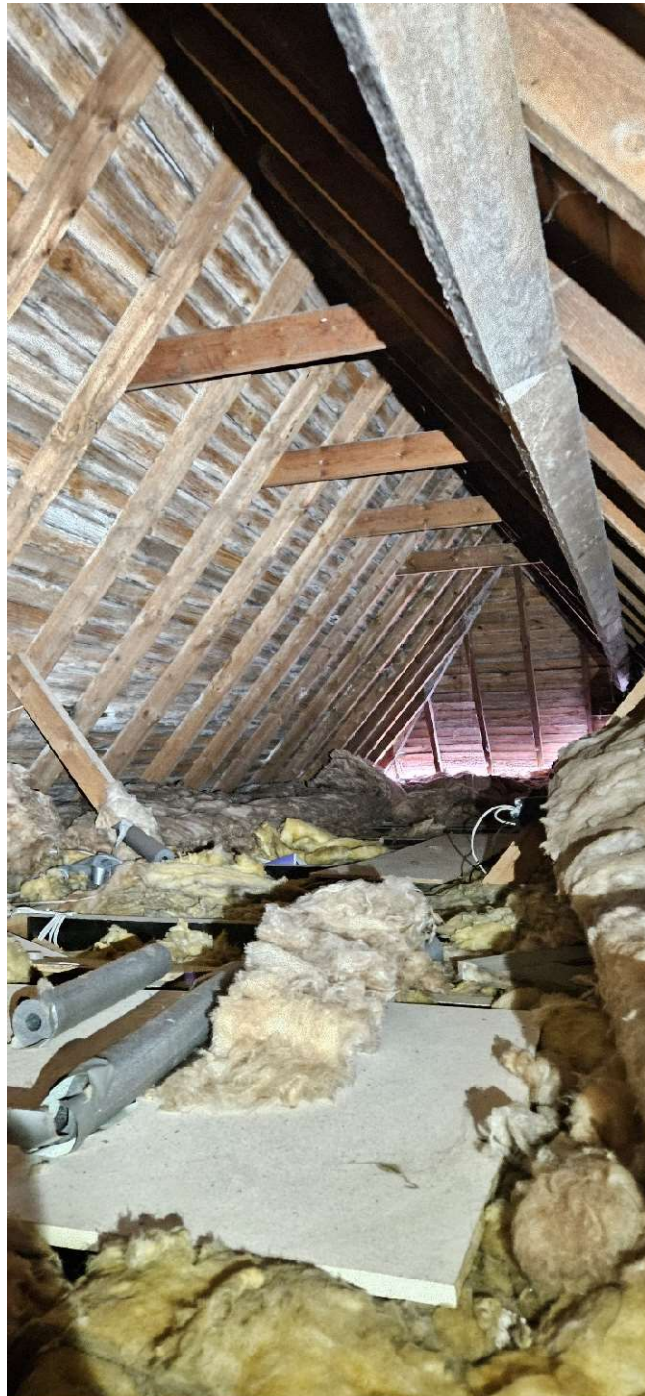
Photo 8 – Loft void facing east demonstrating light ingress
