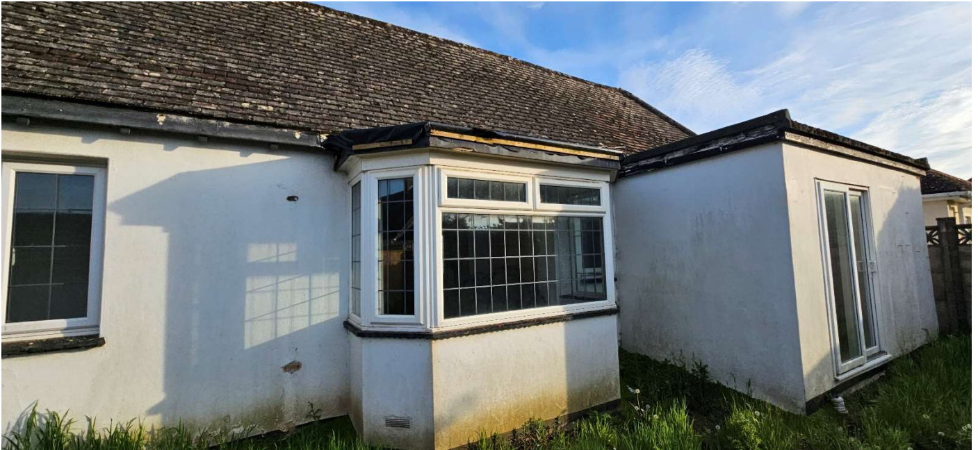
Photo 3 – North elevation of the building
