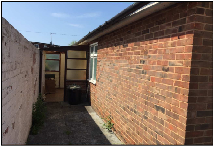
View looking South from the North Eastern corner of the house
