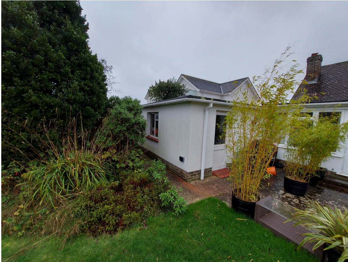
Garage rear and north elevation.
