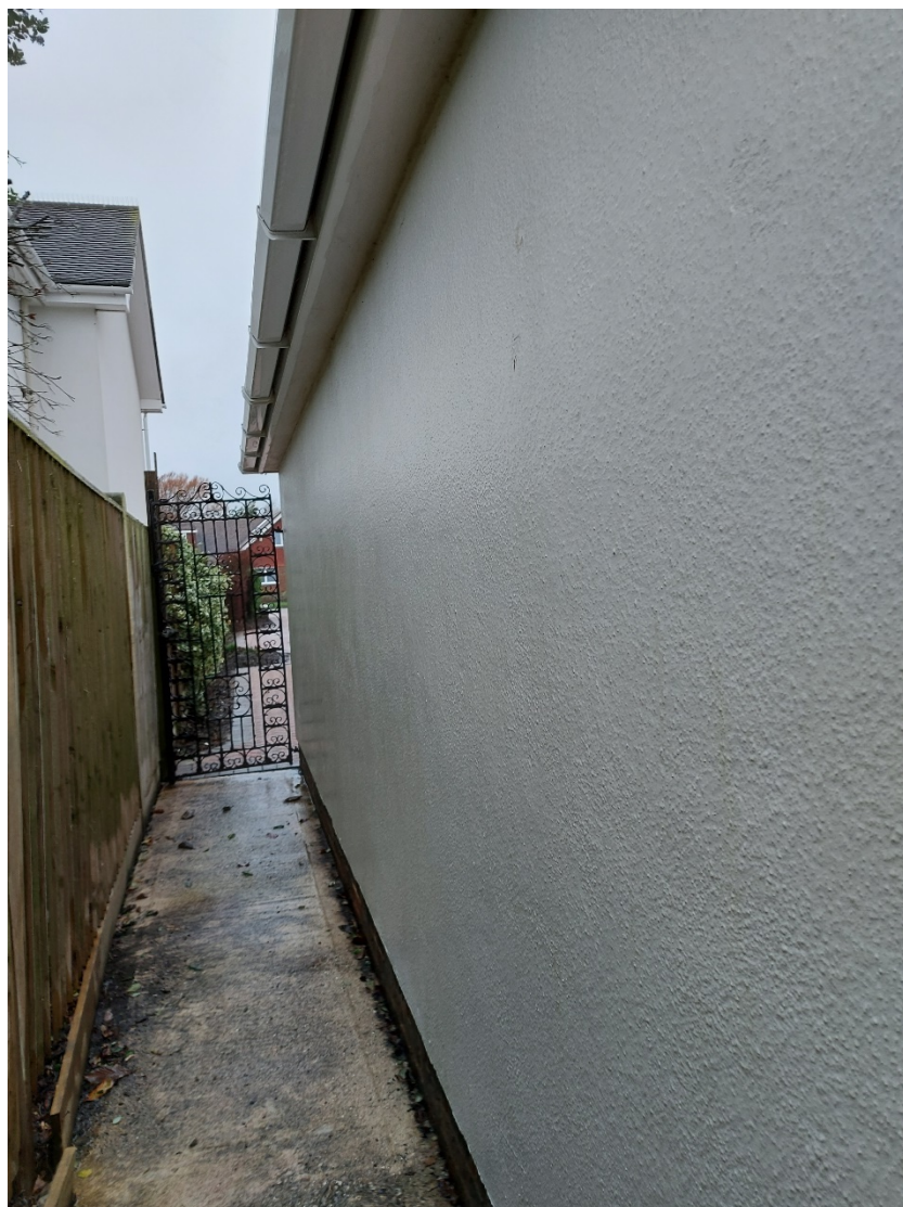
Garage south elevation wall.
