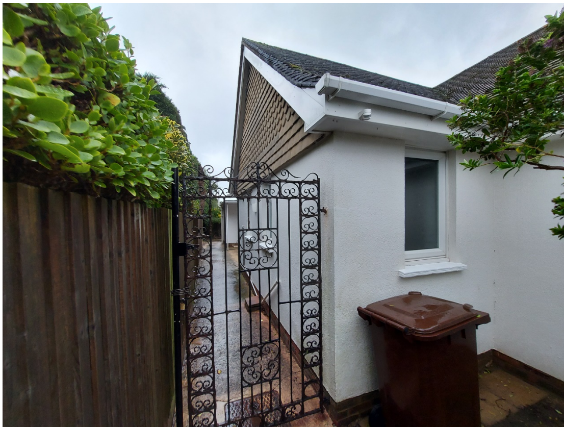
Northern gable end wall.
