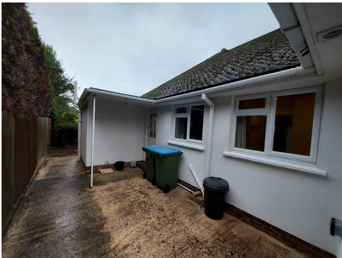
North elevation to the rear.
