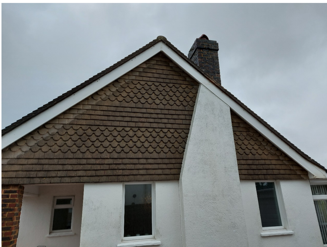
Southern gable end wall.
